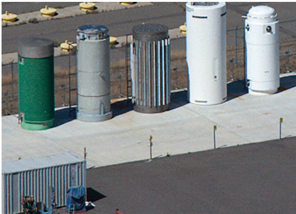
Dry casks of spent nuclear fuel on a storage pad.
